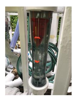
One early morning in May 2019, the A2A and Pipecare teams isolated the first pipe section of a total of three to be treated. Measurements taken by the see-through rotameter were shown to be compatible with the utility's readings of a substantial **8,900** litre/hour (2.5 litres-per-second) aggregate leakage in a 440 meter long section that was assigned by A2A for treatment.
